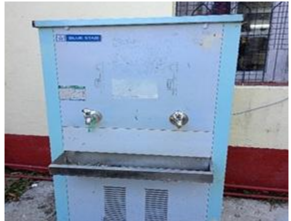
Push Taps Installed to Conserve Water
