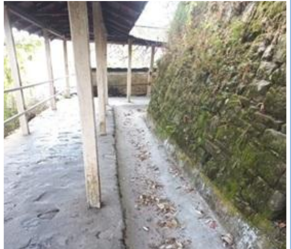
Storm Water Drainage
