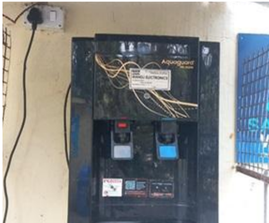
Water Filtration Unit
